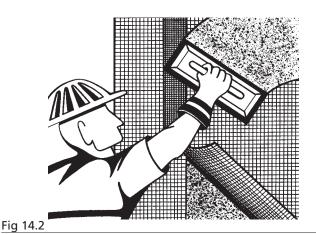
This method keeps the mesh laying flat, ensuring consistent embedment into the basecoat (Figure 14.2). Additional basecoat material may be added to the surface of the fresh basecoat in order to ensure proper embedment of the mesh.
